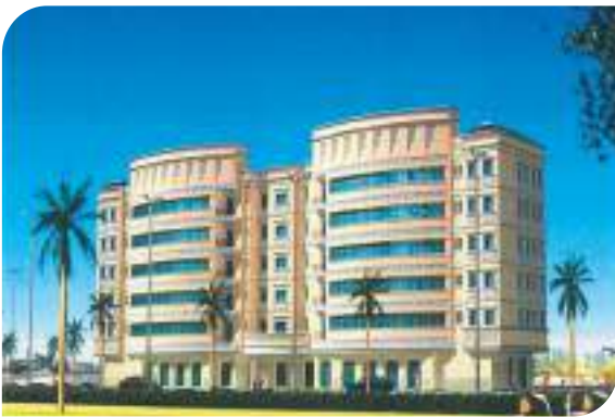
Residential & Commercial Building, Abu Dhabi
