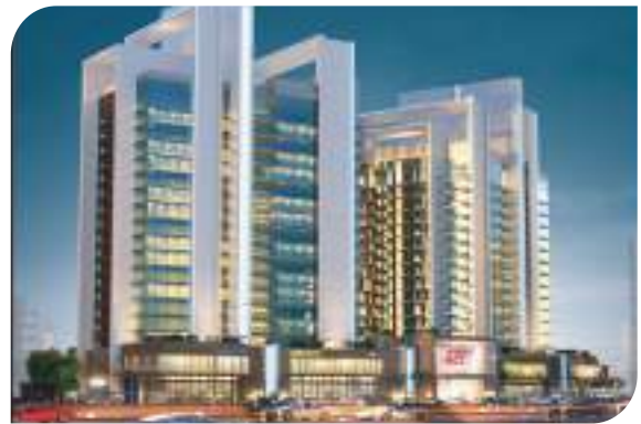
Danet Twin Tower, Abu Dhabi
